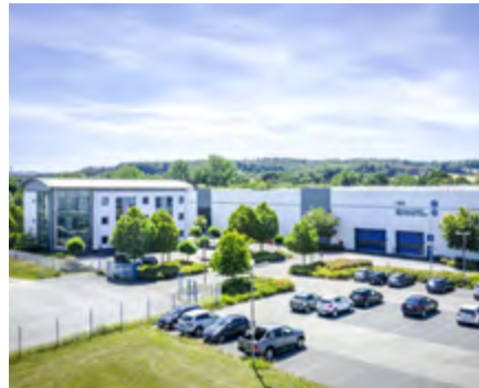
OKS Iserlohn plant (Germany)
