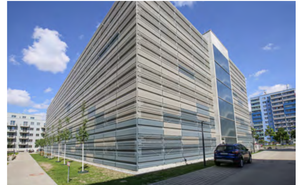
Split-level car park in Berlin with a design that blends into its surroundings
