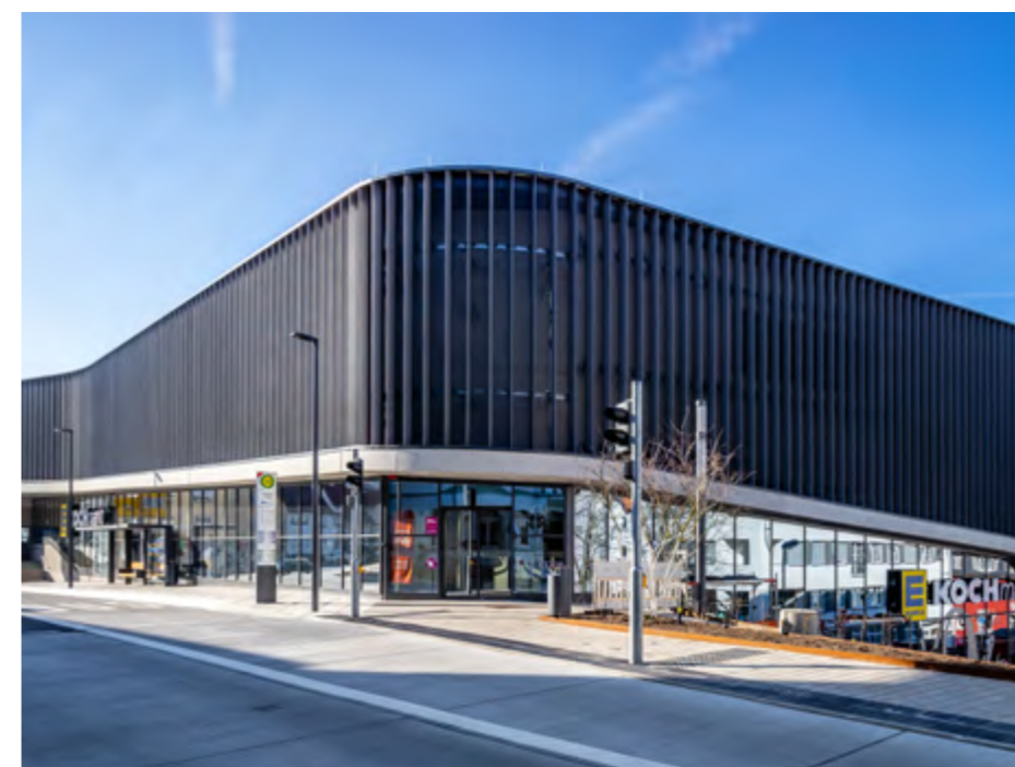
SCHÄFER Perforated Metal supplied 1,250 square metres of aluminium perforated sheets for the new EDEKA building in Albstadt
