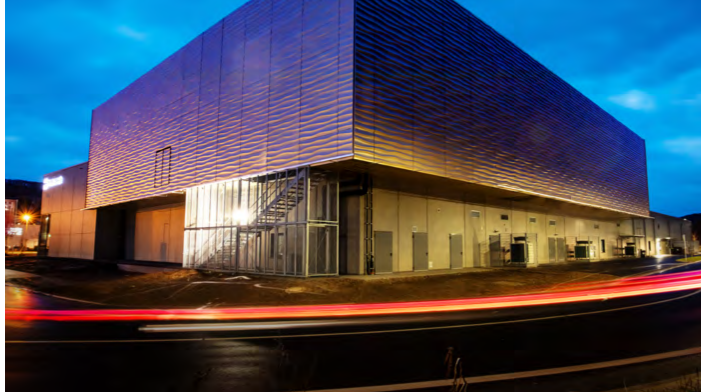
The H+ Carré shopping centre in Herdorf, including the "Herdorf water wave" 3D façade made of perforated sheets
