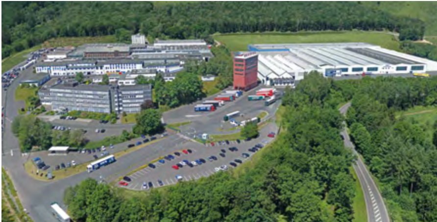
Head office and plant, Neunkirchen (Germany)
