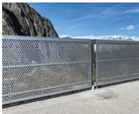
Dam wall with railing made of perforated sheeting at Lake Albigna
