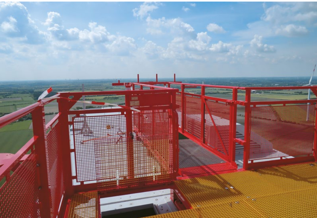
Assembling a helihoist at a lofty height
