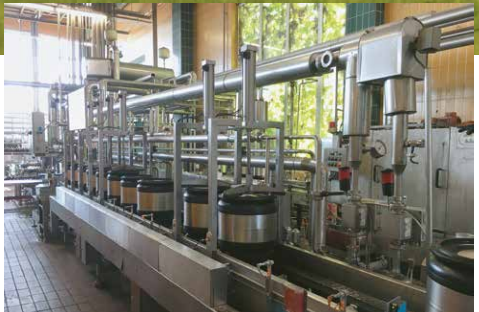
ECO KEGs from SCHÄFER Container Systems on the Ayinger filling line
